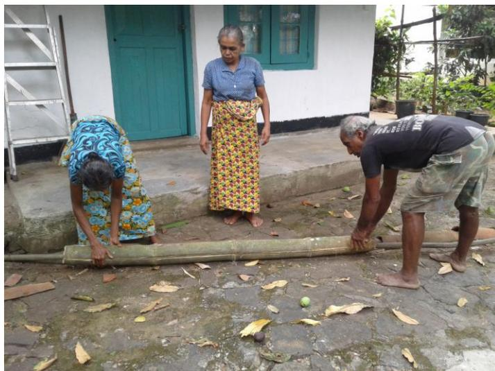
PVC pipe being encased in giant bamboo
